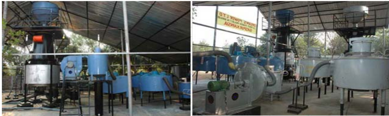
Figure 2: Front face of power plant
